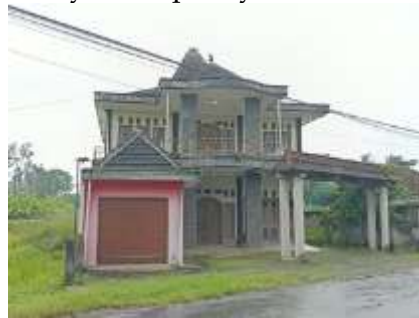
Figure 10. Construction of a Regol Gate in a Private Residence
